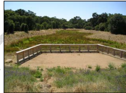
Detention and Filtration Wetland area
