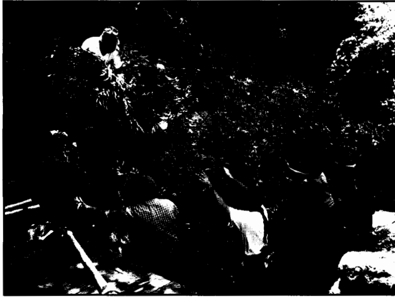
UCC staff lead a demonstration project on Codornices Creek in Berkeley. Local homeowners learned how to install soil bioengineering methods to prevent erosion, such as the brush mattress seen here.
